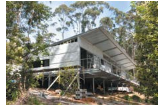
Bushfire resilient home under construction, using flame resistant sarking. Source: Ian Weir
