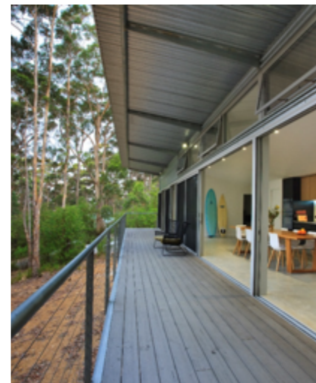
Example of deck well maintained, clear of clutter. Source: Andrew Halsall
