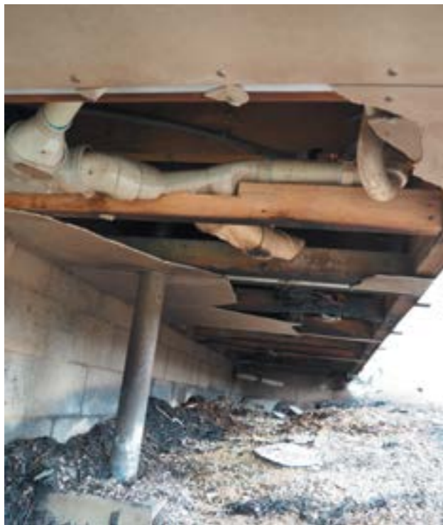
Underfloor damage caused by burning garden bed, suppressed by fire agency before it burnt into the house. Source: CSIRO
