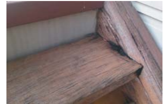
Ember attack in re-entrant corners. Source: CSIRO
