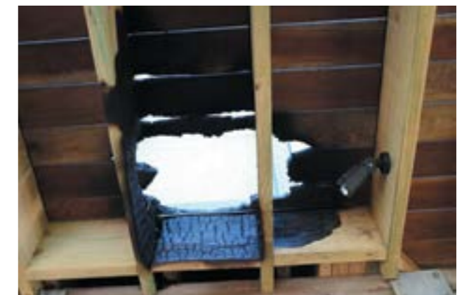
Damaged deck by ember attack (potential issues with exit path).
