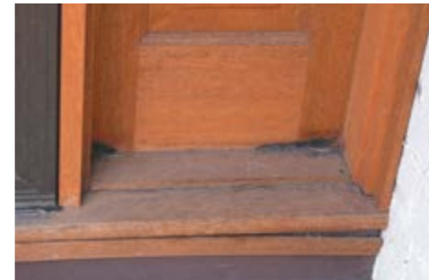
Embers attack in re-entrant corners. Source: CSIRO
