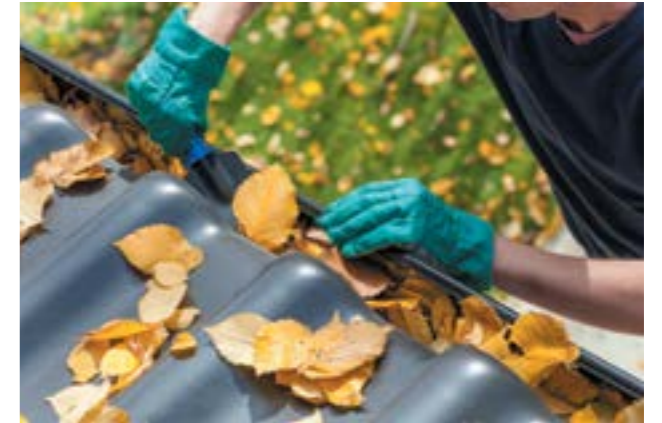
Regularly clean debris from your gutters.
