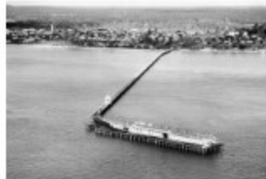
The pier was originally used to export coal and sugar on cargo trains. (Supplied: FCRC)
