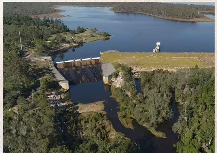
Aerial image of Lenthalls Dam and spillway.
