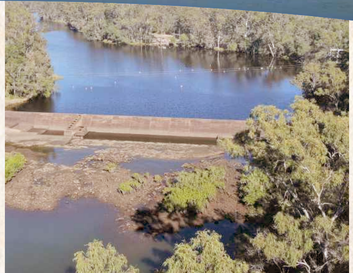
Burrum Weir No.1 showing freshwater storage above the weir and tidal zone below.
