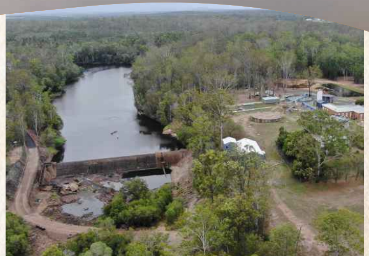
Aerial image of Teddington Water Treatment Plant and Teddington Weir.
