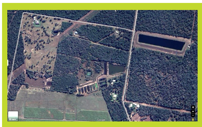
View of recycled water retention basin on Vanderwolf Road, Bunya Creek.
