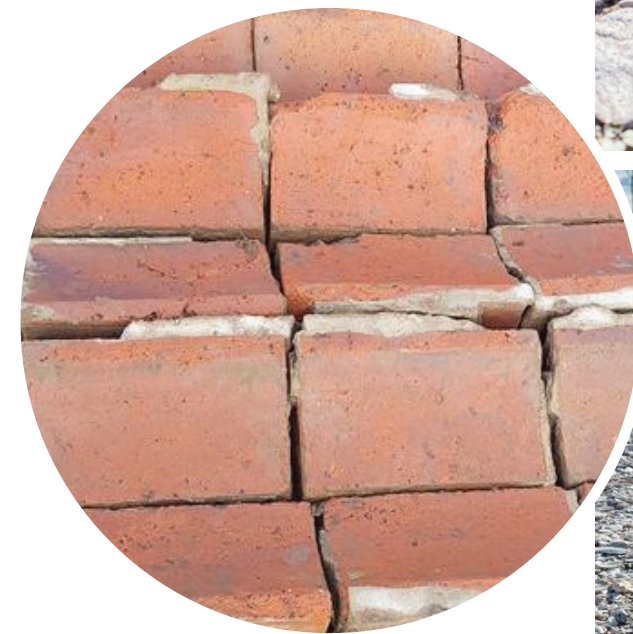
The recovered clay bricks
