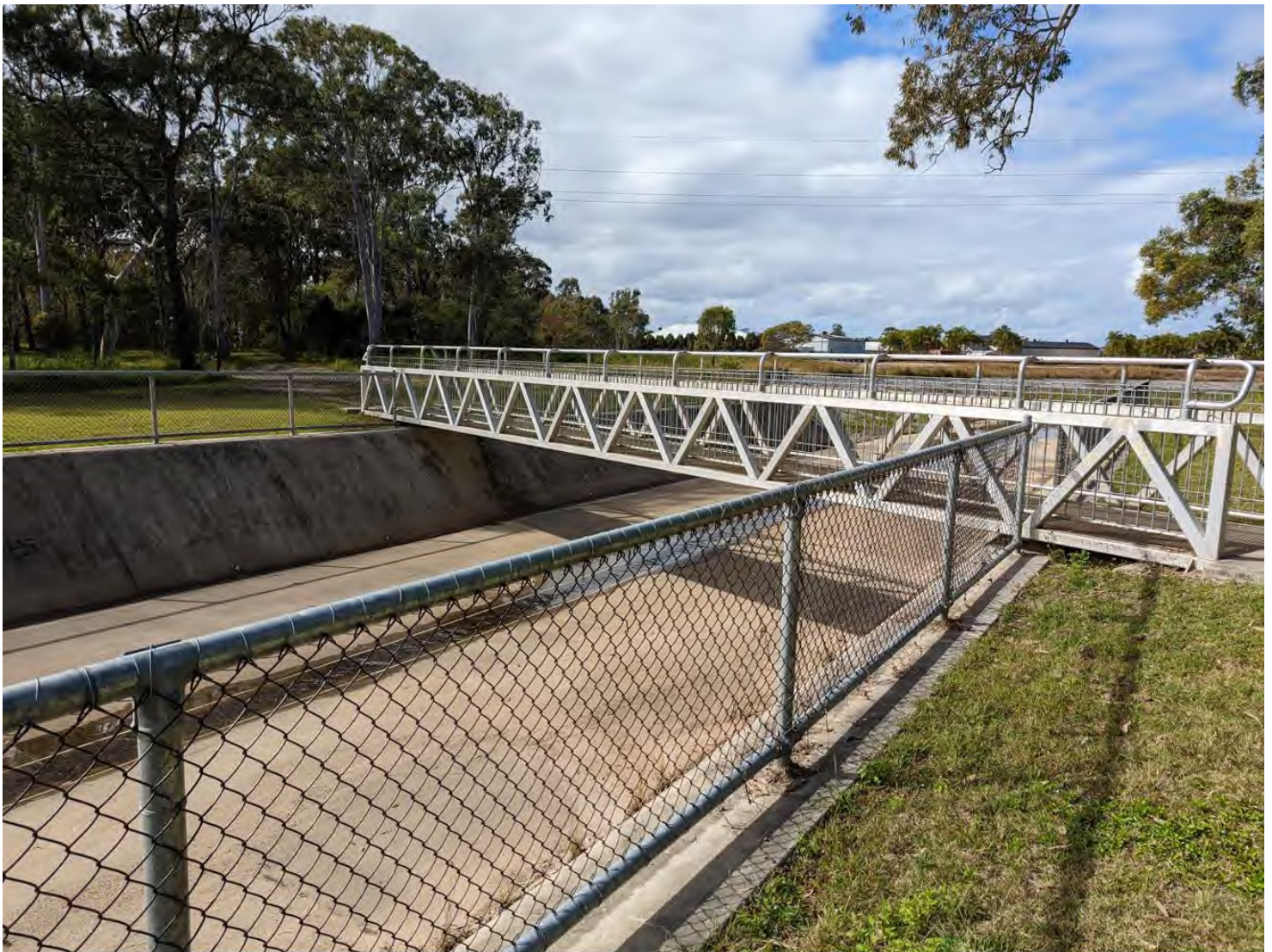
Figure 6-1 Doolong Road Pedestrian Bridge
