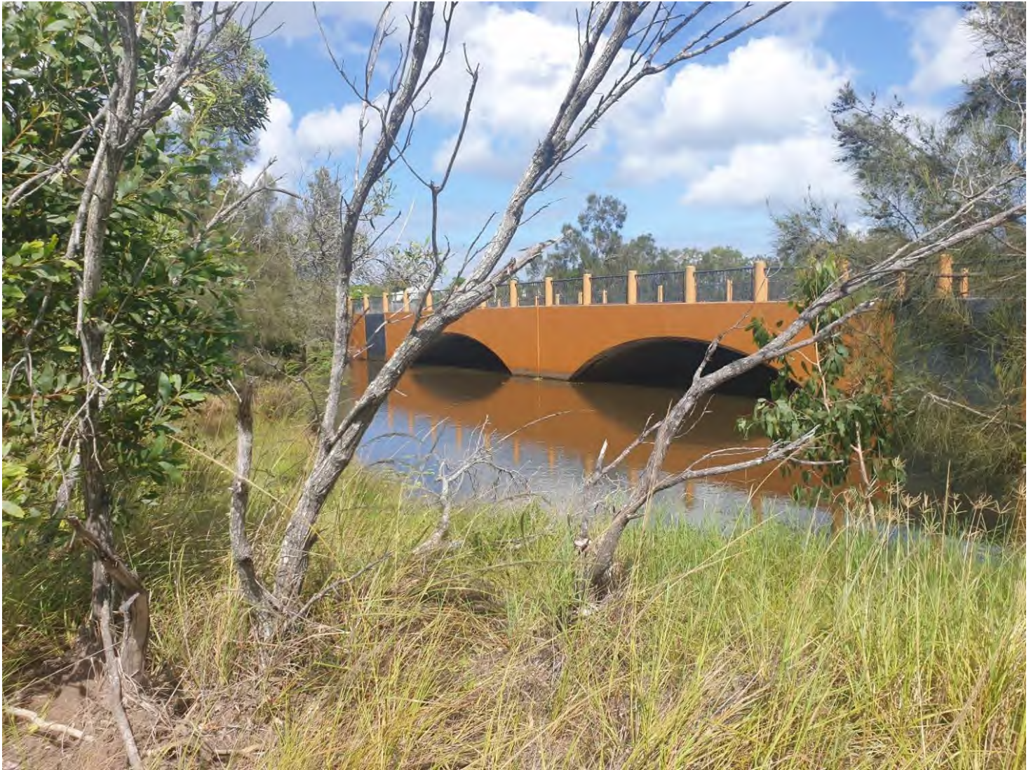
Figure 6-3 Endeavour Road Bridge
