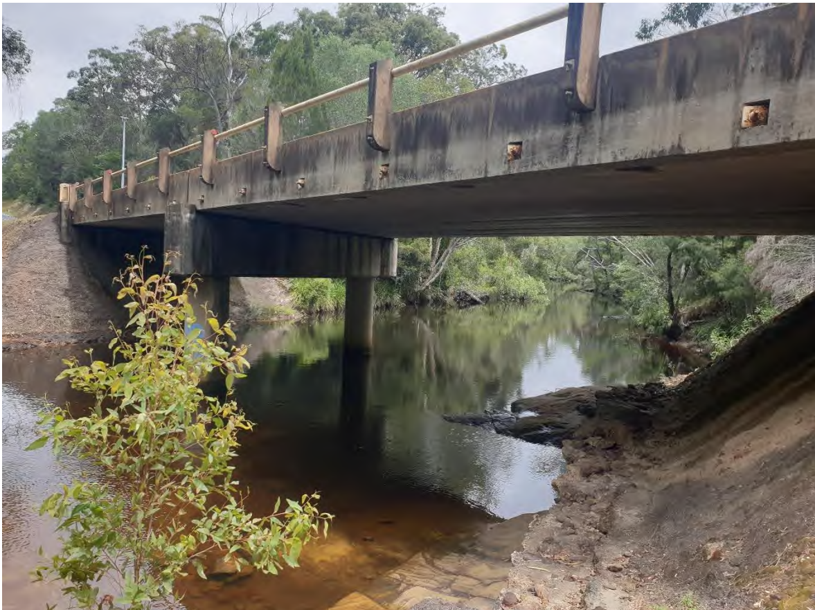
Figure 6-1 Poona Creek Bridge
