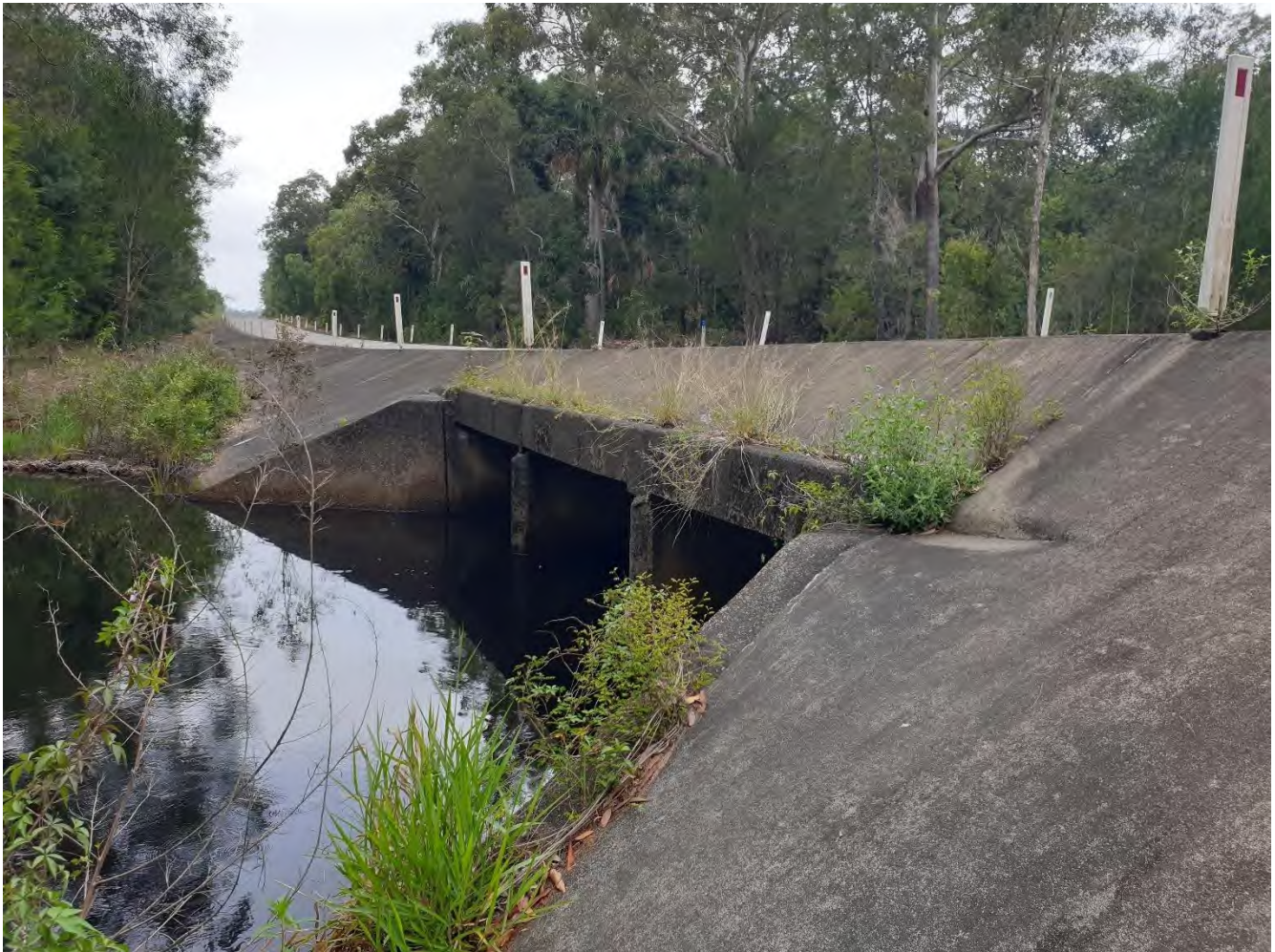
Figure 13-1 Scrubby Creek Causeway and Culverts
