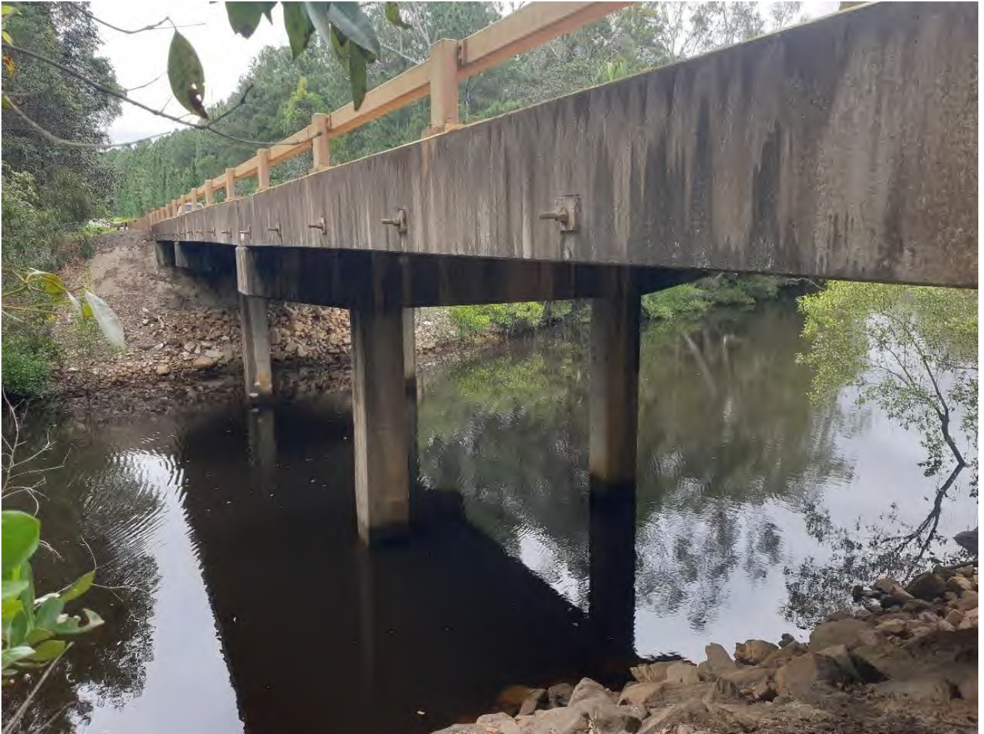
Figure 6-3 Big Tuan Creek Road Bridge
