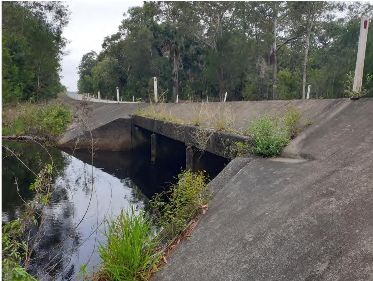
Figure 12-1 Scrubby Creek Causeway and Culverts
