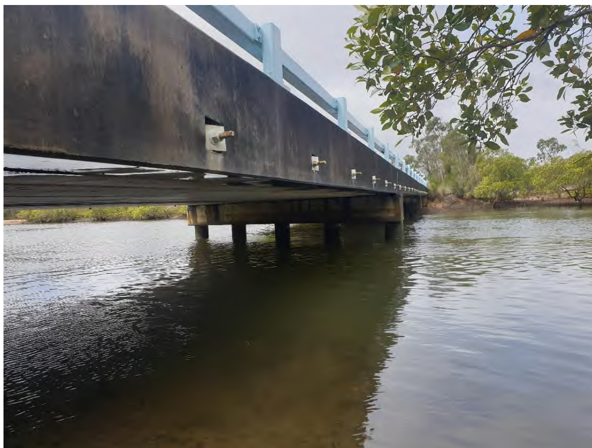
Figure 6-2 Wilkinson Road Bridge
