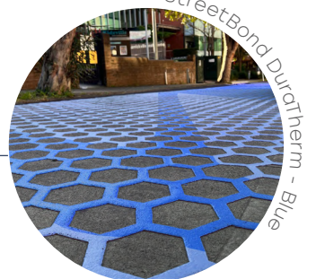
Shared Zone StreetBond on Asphalt Detail
