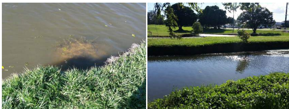
Figure 4-3 Localised edge erosion occurring adjacent to the golf course near the inlet to Ululah Lagoon.
