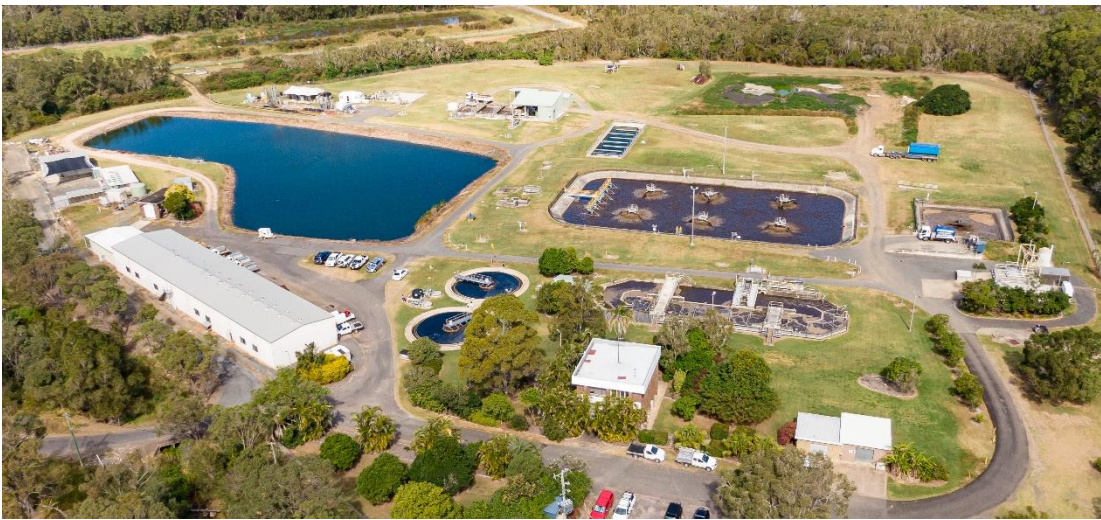
Pulgul Sewage Treatment Plant
