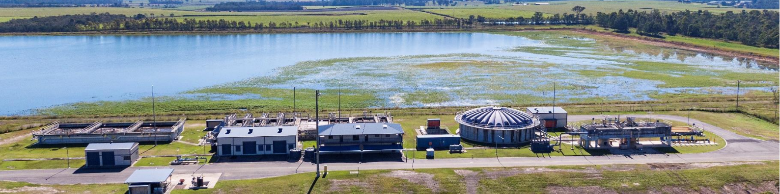
Nikenbah Sewage Treatment Plant
