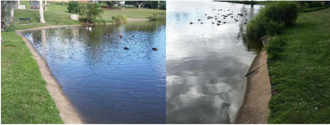
Figure 4-1 Concrete revetment in the SE corner of Ululah Lagoon: a) Main section, and b) Collapsed section towards the northern end.
