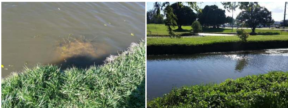
Figure 4-3 Localised edge erosion occurring adjacent to the golf course near the inlet to Ululah Lagoon.
